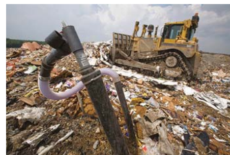
FIGURE 1.1.15 Pipes buried in this rubbish tip collect biogas.
