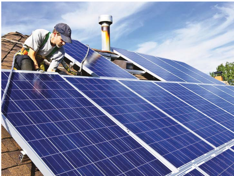
FIGURE 1.2.1 Commercial solar cells convert solar energy to electrical energy with an efficiency of 12–18%.
